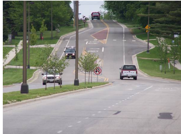
Photo 9.1: Lacy Road in front of City Hall
