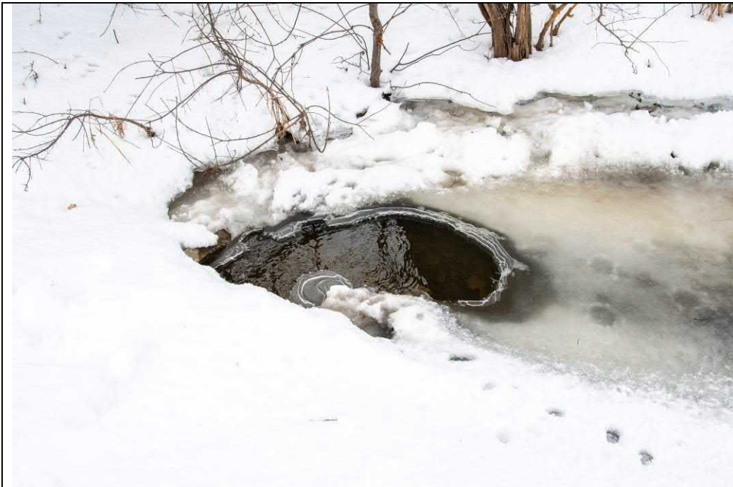
ACTIVE FLOW THROUGH CULVERT AT CUSICK PARKWAY
