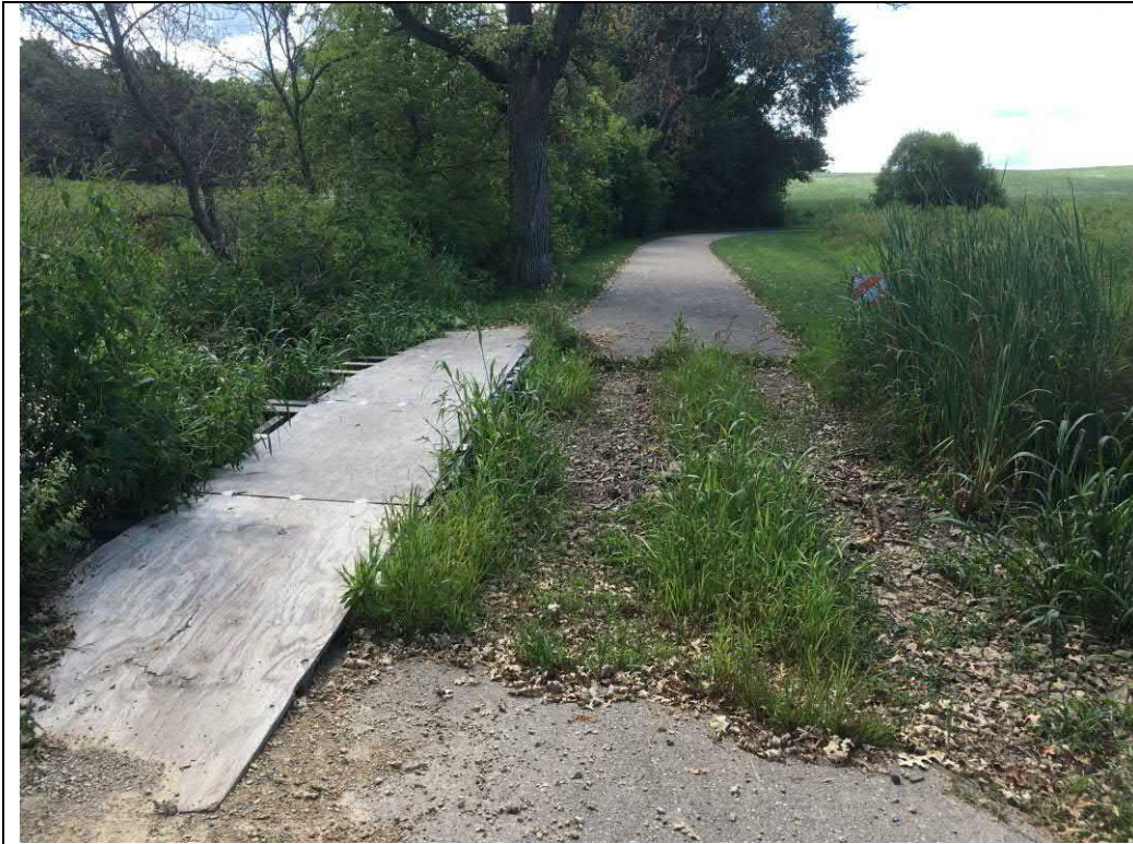
ROTARY TRAIL CROSSING, DRY WITH NO SURFACE WATER NEARBY.
