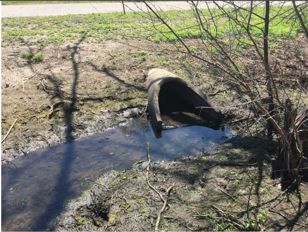
LOOKING EAST AT CULVERT UNDERNEATH CUSICK PARKWAY, ~0.3 CFS
