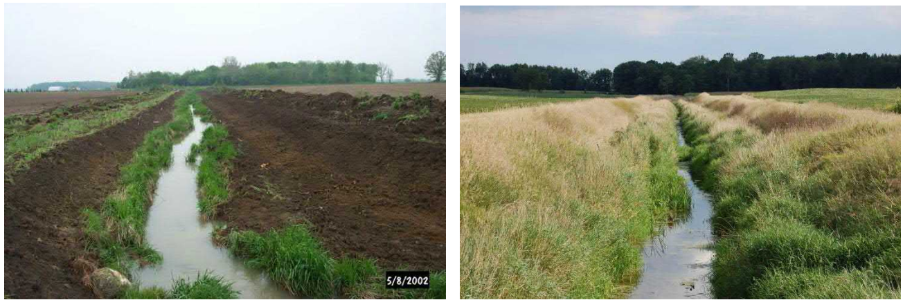
Figure 18. Typical 2-stage ditch during and after construction.
