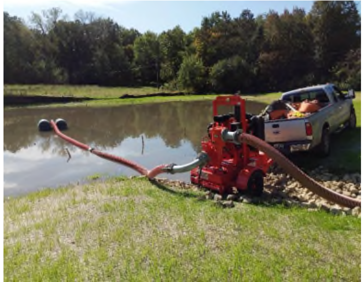
Figure 2. Second Pumping Setup
