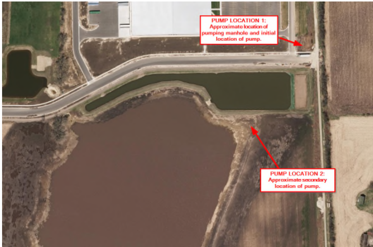
Figure 1. Pump Initial and Secondary Pump Locations
