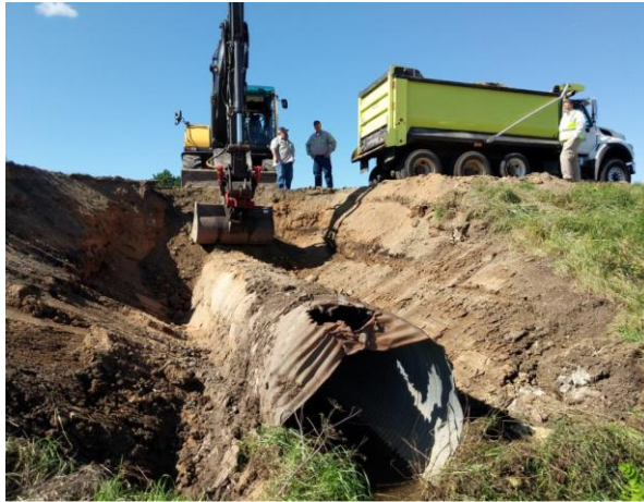
Repairing a corroded culvert
