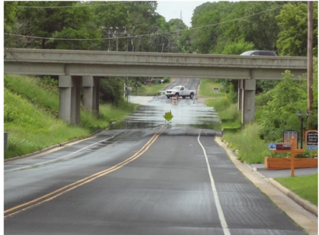
Fitchrona Road, looking south to 18/151, photo taken June 26, 2013
