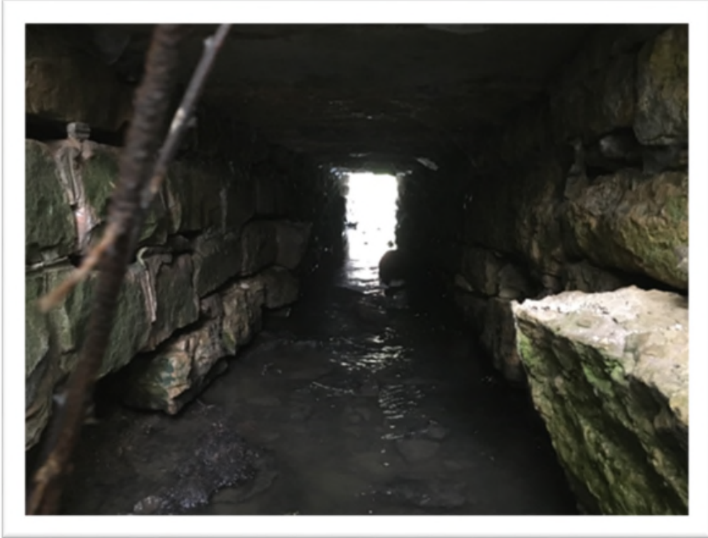
Existing Railroad Culvert 3-ft x 3.5-ft
