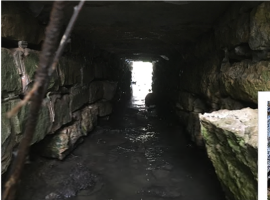
Existing Railroad Culvert 3-ft x 3.5-ft
