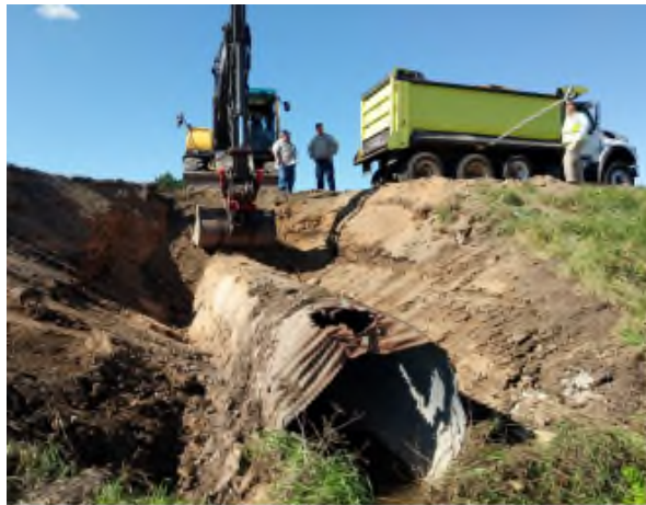
Repairing a corroded culvert
