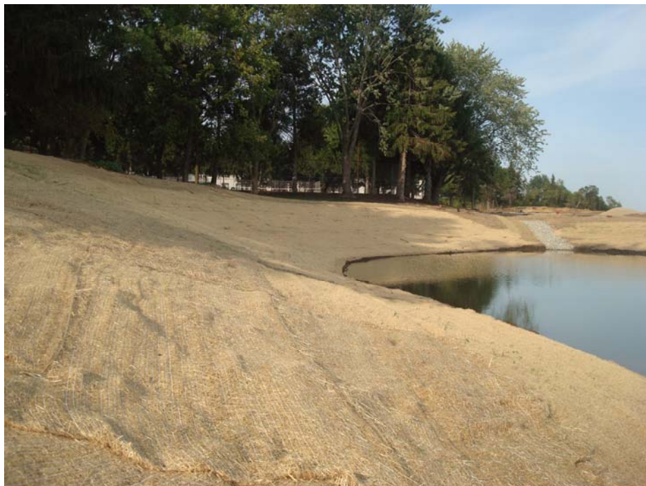
Views of the erosion matting and constructed pond on August 23, 2012
