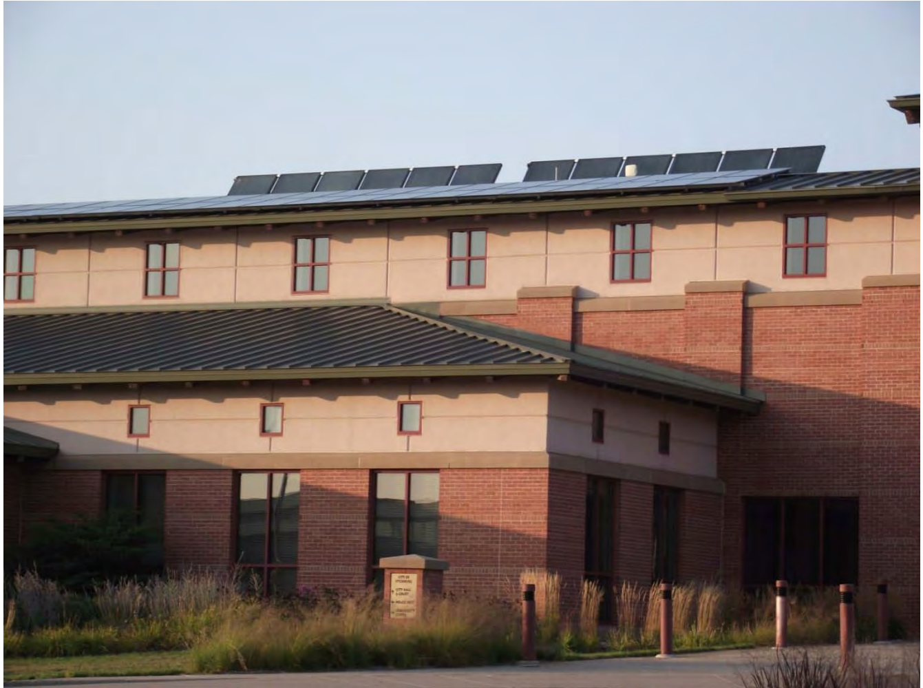
Solar photovoltaic and solar thermal panels on City Hall roof top
