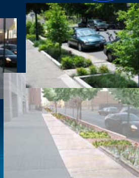
AFTER: Madison Avenue with Stormwater Planters
