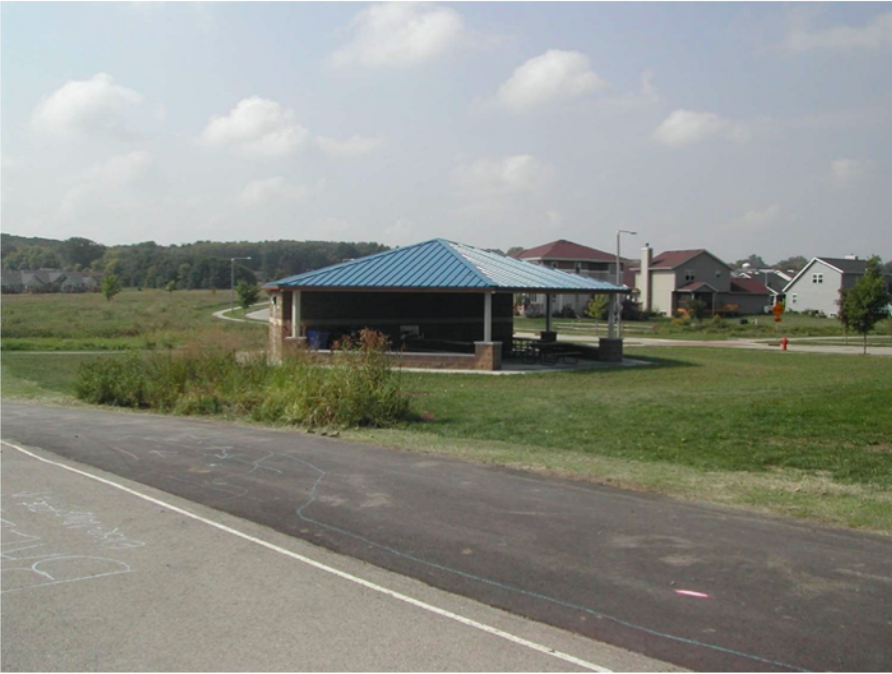
Swan Creek shelter with bathrooms – 2008 construction = $172,251
