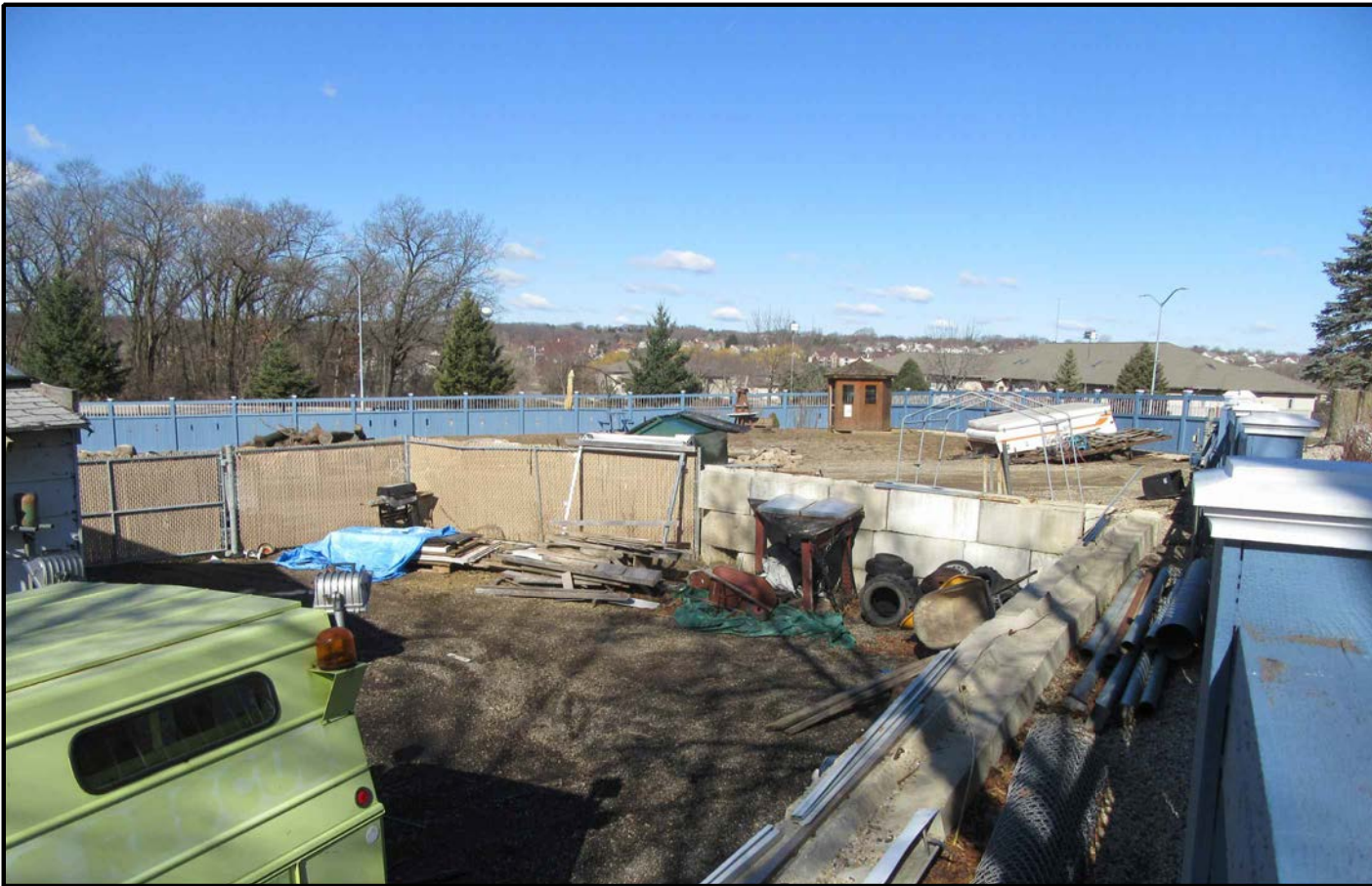
SITE OVERVIEW LOOKING NORTH
