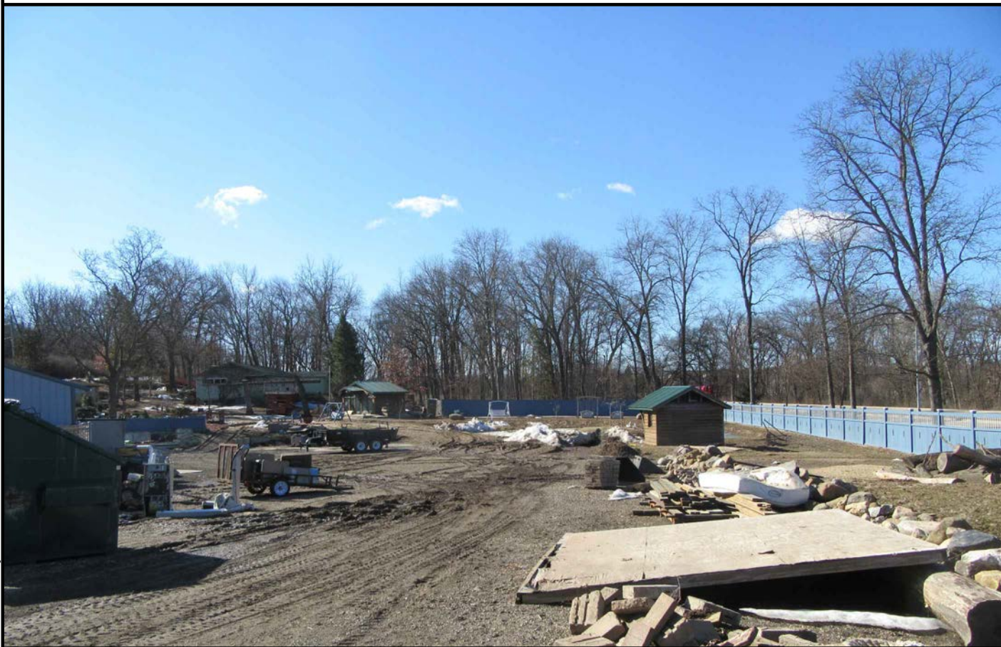
GRAVEL ACCESS DRIVE LOOKING SOUTHWEST
