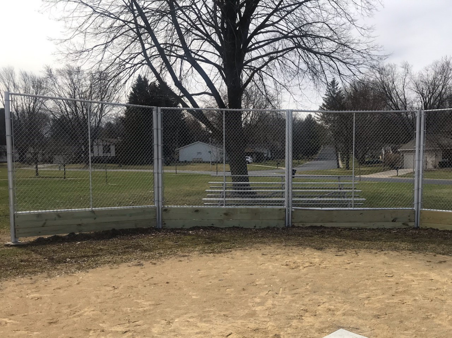
Tower Hill Park ballfield backstop repair.
