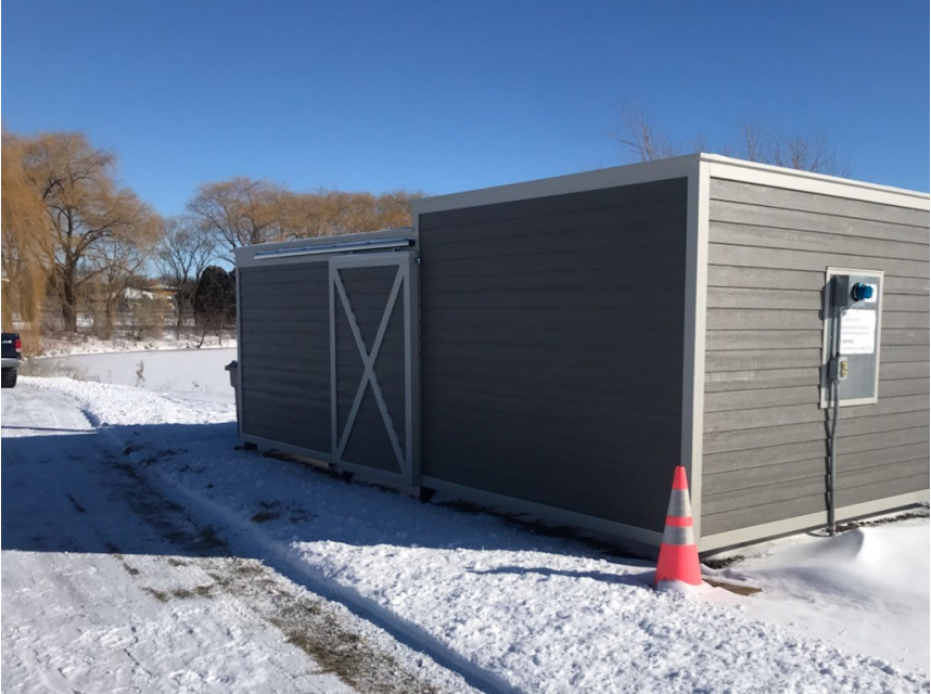
New Utility encloser at McKee Farms Park
