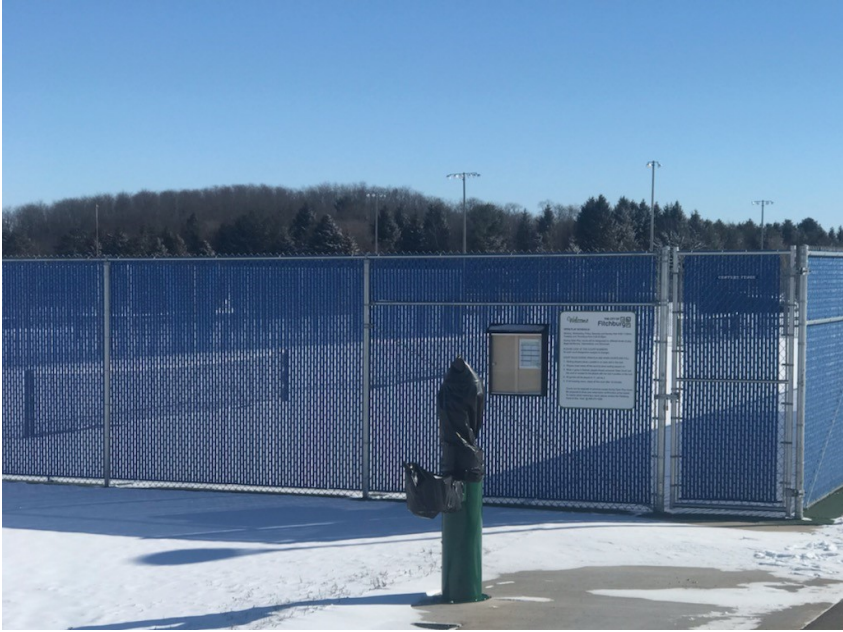
McGaw Park pickleball path lighting, drinking fountain, and slats in fence to reduce wind
