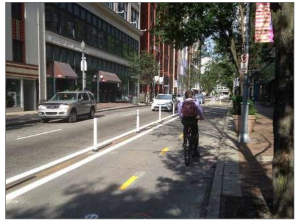
A painted buffer and bollards physically separate bicyclists using the two-way protected bicycle lane from motor vehicle traffic.
