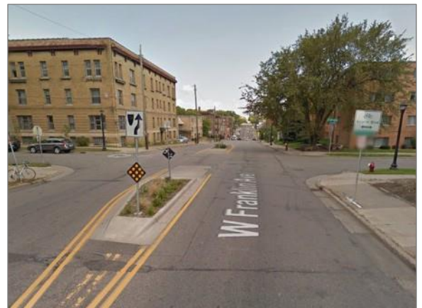
A median refuge at the intersection of Franklin Avenue and Bryant Avenue S (a Neighborhood Slow Street) in Minneapolis makes it easier for people walking and bicycling to cross Franklin Avenue W.
